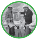
Charles Bronfman, Toronto Mayor Philip Givens and TD President & CEO Allen Lambert on top of steel structure of TD Tower at the "topping off" ceremony, Toronto Dominion Centre, April 14, 1966 TD Bank Group Archives 77-240-10 Ron Vickers Photography 9860-13
