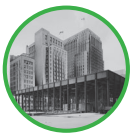
Banking Pavilion under Construction, Toronto Dominion Centre, August 1967 TD Bank Group Archives P10-0158 Panda & Associates 67203-11
