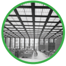
Banking Pavilion Interior, Toronto Dominion Centre, 1970 TD Bank Group Archives 77-247-22
